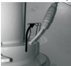
Diagram 4 Push LED connectors into ceiling
